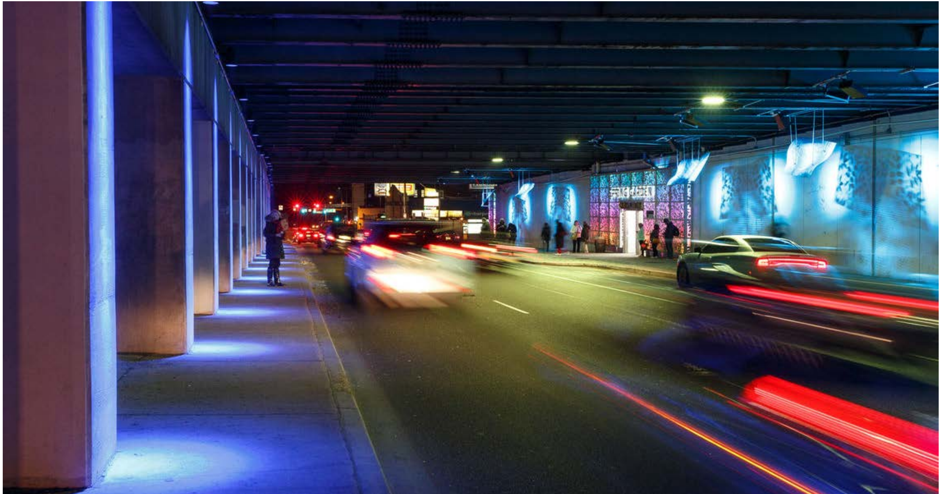
Median Columns with Color Wash
